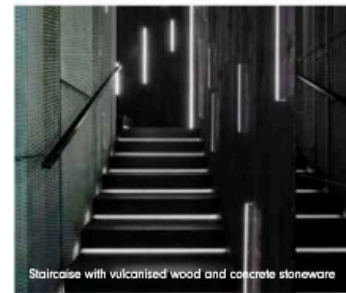
Staircase with vulcanised wood and concrete stoneware
